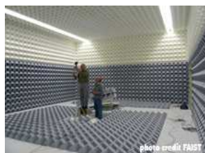
absorbing lining based on wedges for an anechoic room (electronic industry)
